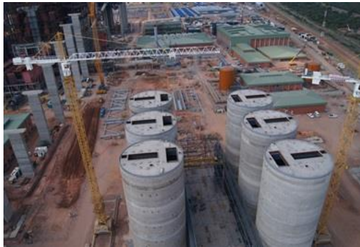
Figure 21 – Medupi Construction Site
