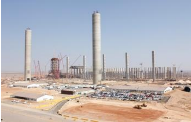
Figure 22 – Kusile Construction Site
