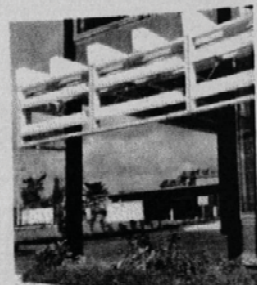
39. Timber framed house
