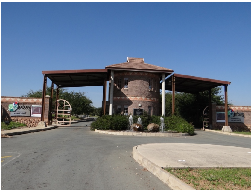
Figures 6.10: A double-storey administrative building at Waterval Cemetery
