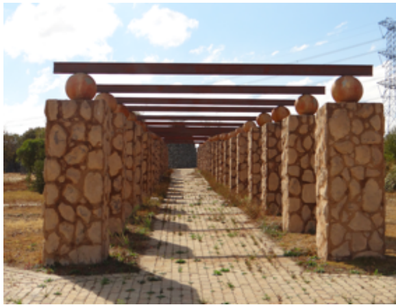
Photograph 0.1: Pathway leading to the gabion tower
