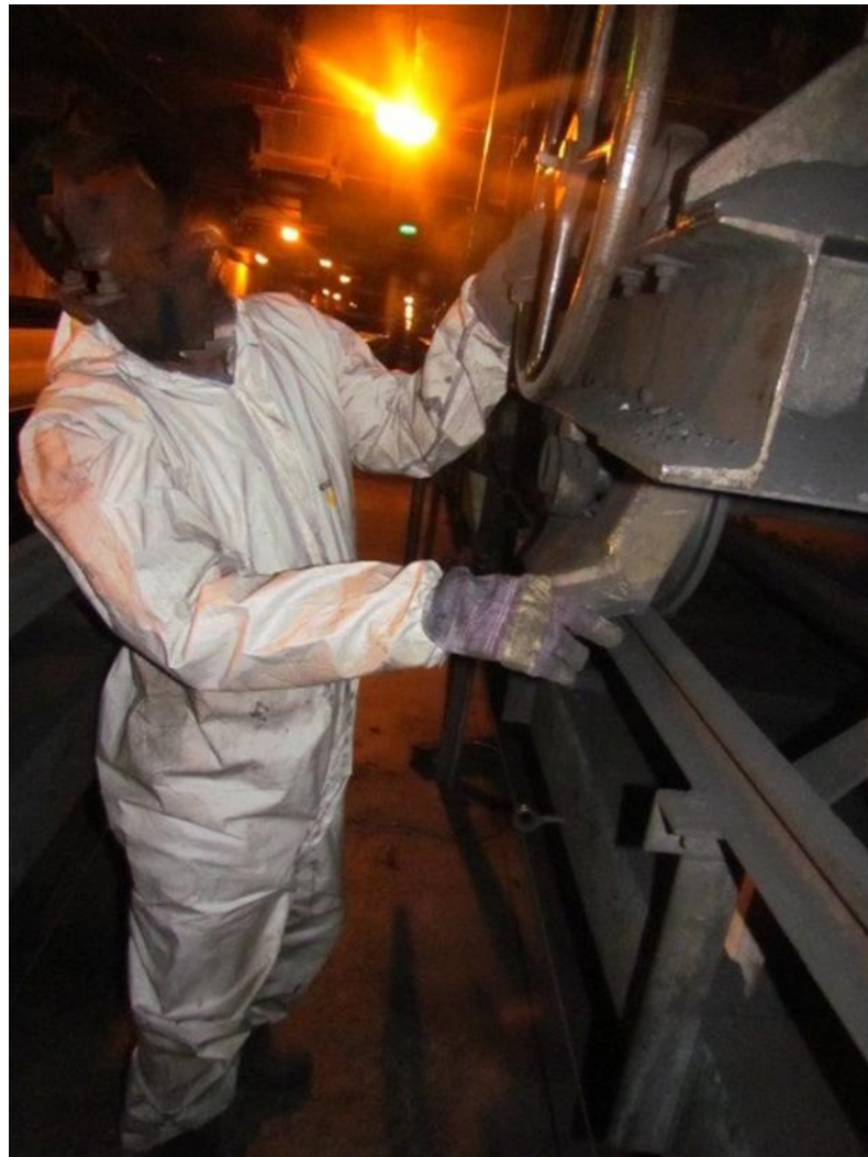
Figure 8: Mechanical Maintenance worker inspecting a fault on the conveyor system
