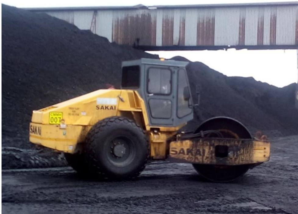
Figure 7: Compactor maintaining road surface for trucks at the coal stock yard
