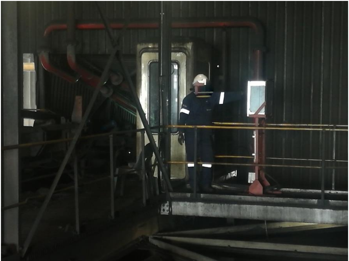
Figure 4: Belt Plant operator at the control panel
