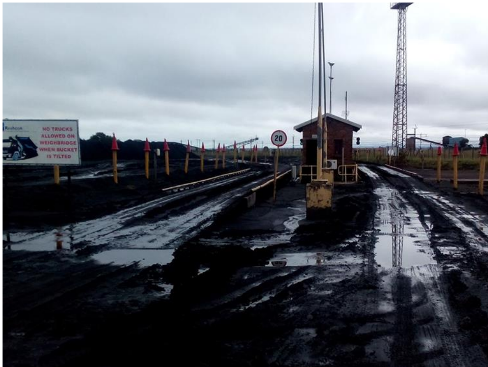
Figure 3: Coal stockyard Weighbridge and Plant operator cubicle
