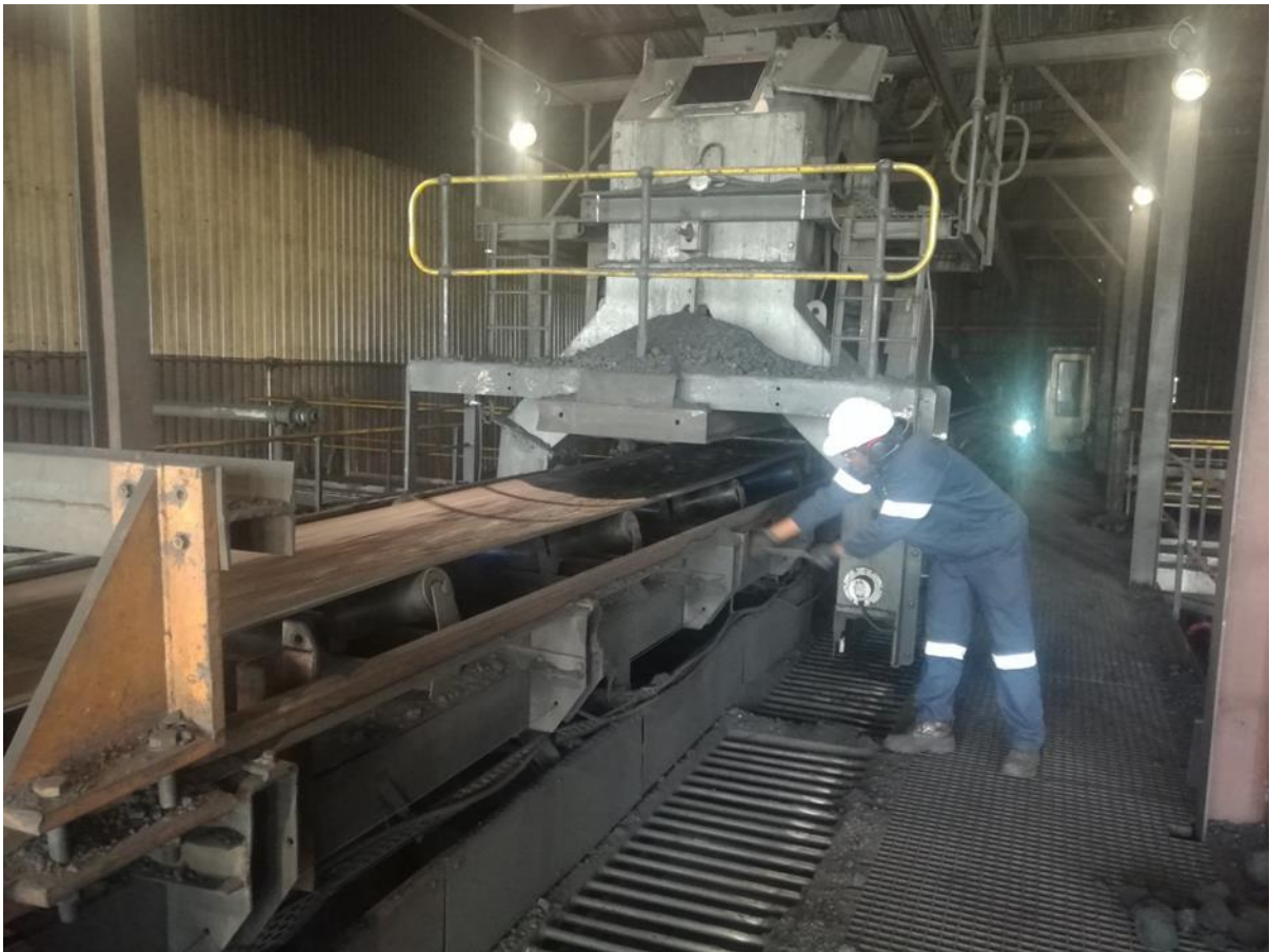
Figure 5: Coaler operating tripper car to load coal bunker
