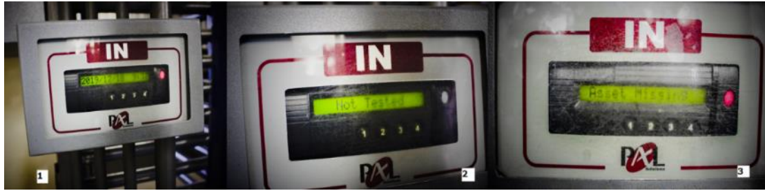
Figure 5.36 T&A Swipe Access Point Message: before miner swipes in (1), after miner swipes with a not tested Virocap Lamp (2), after miner swipes without the assigned Virocap lamp
