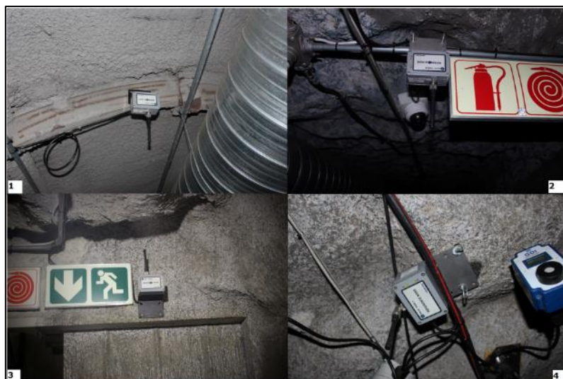
Figure 5.17 Four Minetec Reference Nodes at Different locations in Mock Mine Tunnel
