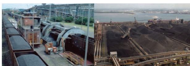
Figure 13—(a) Coal tipplers transferring coal at Richards Bay before (b) being stacked on blending stockpiles
