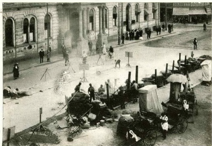
Photo of Asphalt Road being laid by Jenkins & Co., outside G.P.O., Johannesburg
