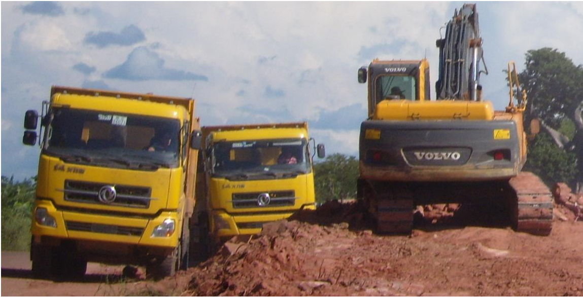
A Chinese construction company enlarging the road that stretches from Dondo to Luanda.
