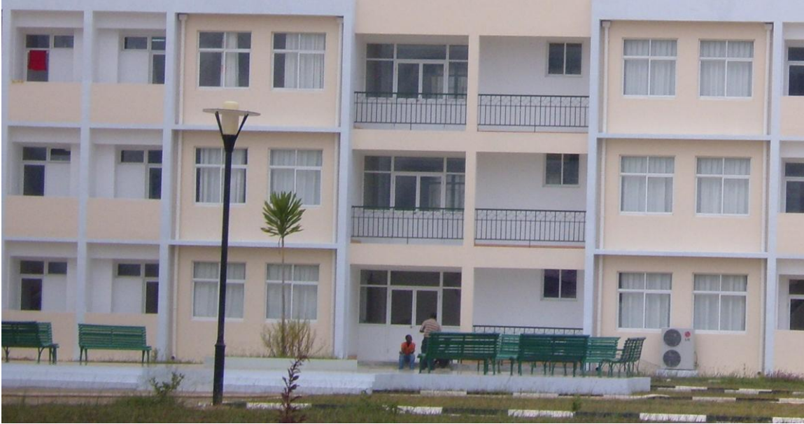
An agricultural college built by a Chinese construction company in the city of Huambo
