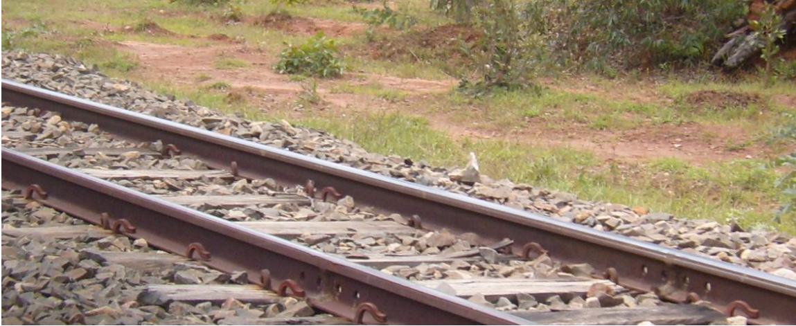
A portion of the railway that stretches from Luau to Lobito rehabilitated by International fund ltd.
