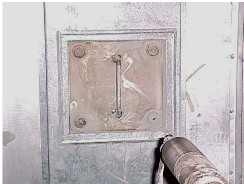
Figure 4.2b: Access hole in boiler wall. Slag probe in the foreground
