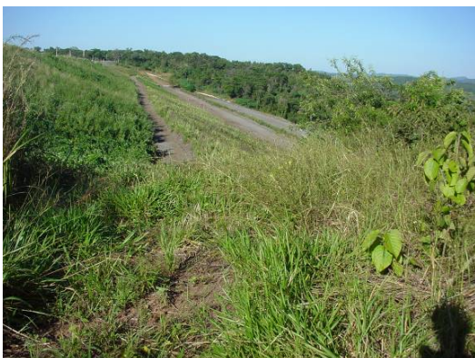
May 2004 – View along the outer face – note the good vegetation establishment.
