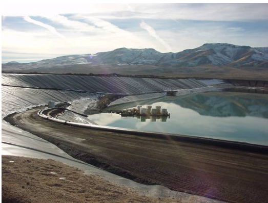
View of the tailings facility – note the liner up the inner face of the impoundment wall.
