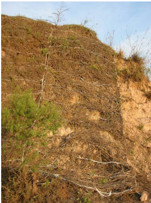
Grass mats on a sandy high wall face. Surprisingly good results are obtained on rocky faces.
