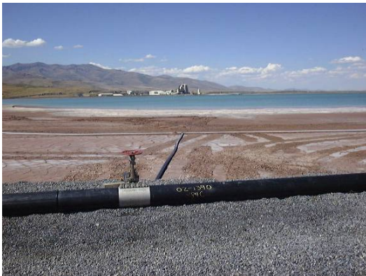
August 1999 – View of relatively short beach caused by large pool. Crest of perimeter wall is in the foreground.
