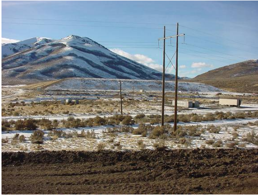
Big Springs tailings facility in December 2000.
