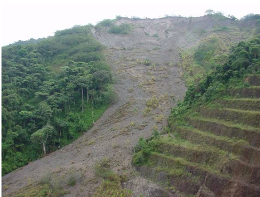
Pit slope failure.
