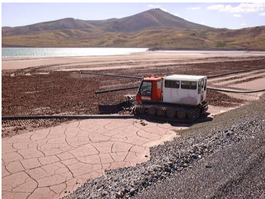
August 1999 – high flotation vehicle on beach. Relocation of beach irrigation infrastructure.
