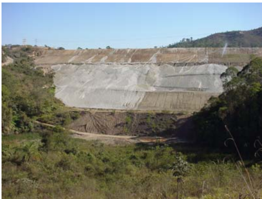
August 2002 - Close-up of impoundment wall at the start of rehabilitation efforts.
