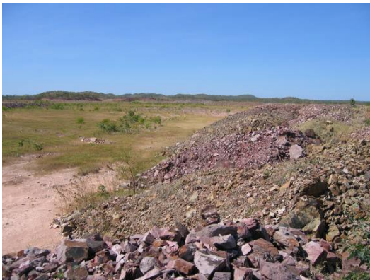
Basin at the point where it meets the crest of the main impoundment wall. Note the waste overburden material used to cap the basin.
