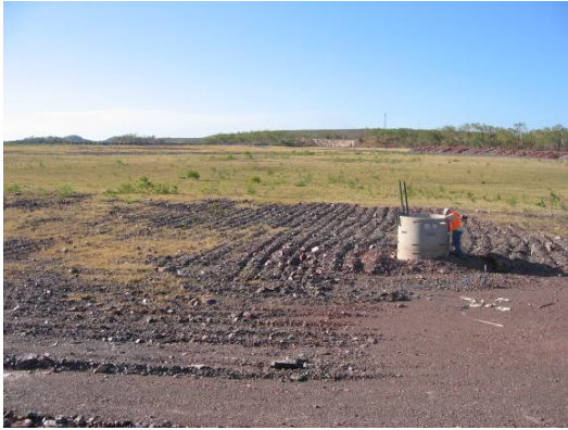
View of tailings facility basin at decant.
