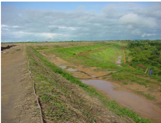
Wet season 2003 – View along the main impoundment wall after rains.
