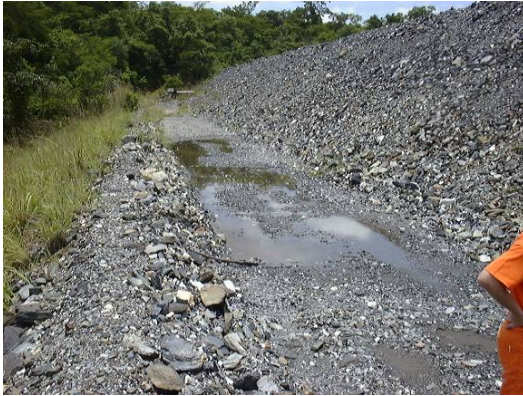
November 2001 – View along bench showing some ponding of storm water after rains.
