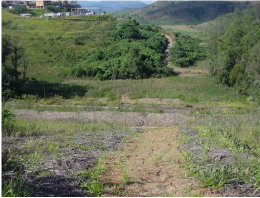
May 2004 - View down face of impoundment wall showing repair of eroded section.
