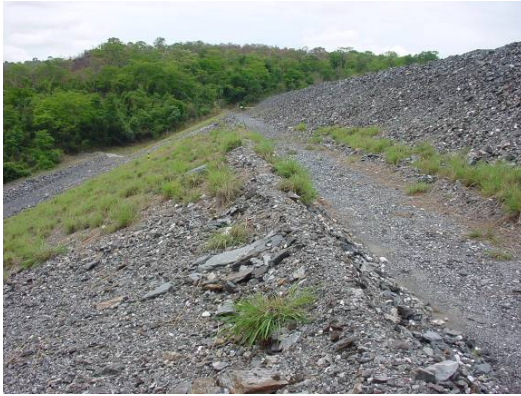
October 2000 – View along bench of main impoundment wall. Note the waste rock cladding with some vegetation growth.
