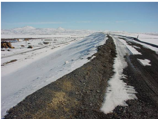
December 2002 – Crest of the impoundment wall.
