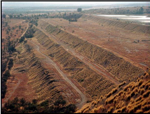
Figure 2.1.1: Tailings deposition behind a cross-valley impoundment formed from mine waste material
