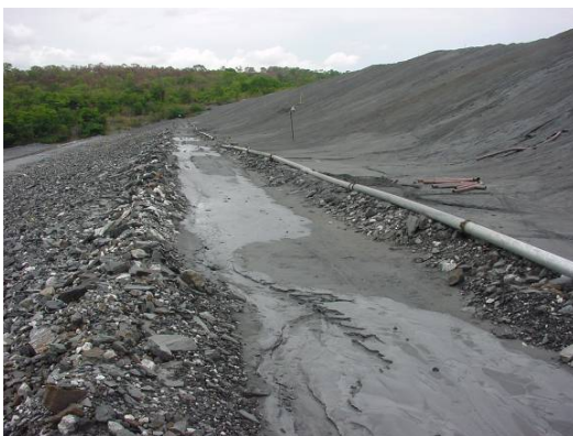
October 2000 – Unclad cycloned material showing some erosion onto the bench.
