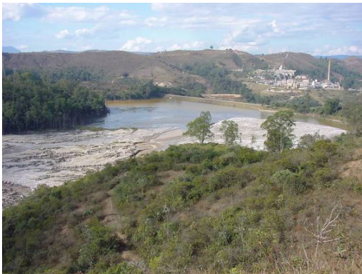
July 2003 - Removal of excess water from the tailings facility basin has resulting in a large area that causes new problems. Note the erosion channels on the dry beach sections.
