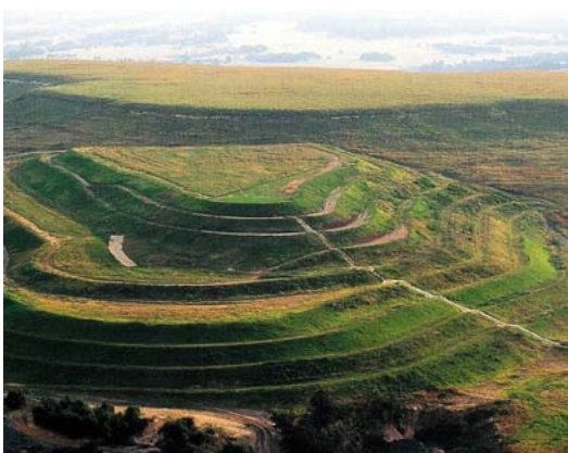
Dump D after rehabilitation:
