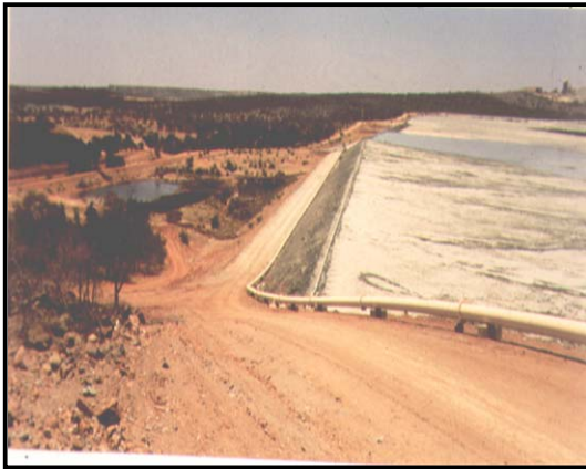
Figure 2.1.3: Tailings disposal via spigot deposition
