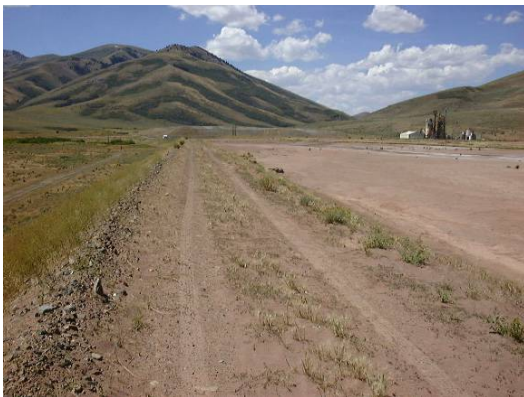
August 1999 – Impoundment wall crest – note the vegetation establishment on the outer face.
