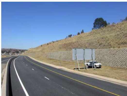
Biotechnical rehabilitation of excavation through a slimes dam.
