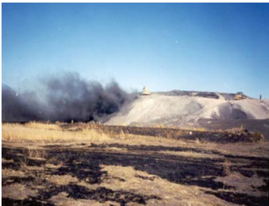
Dump E during rehabilitation works:
