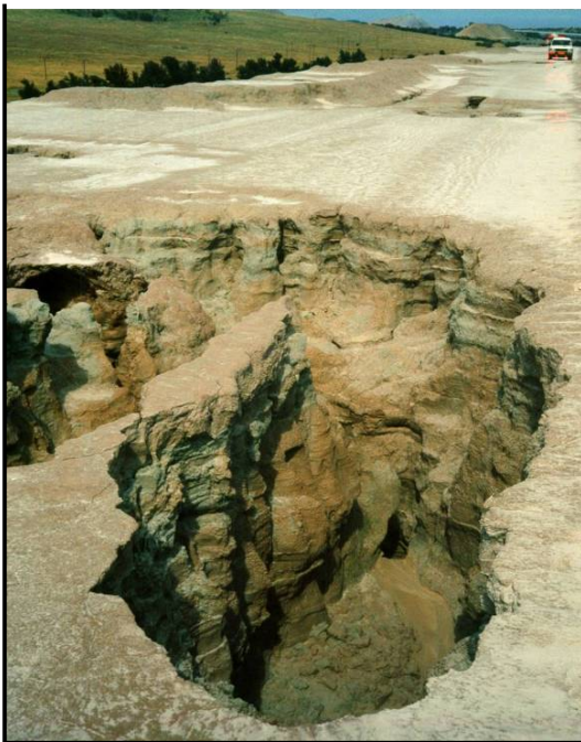
Figure 2.2.5: Erosion caused by water ingress
