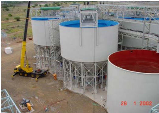
Thickener erection at retreatment plant.
