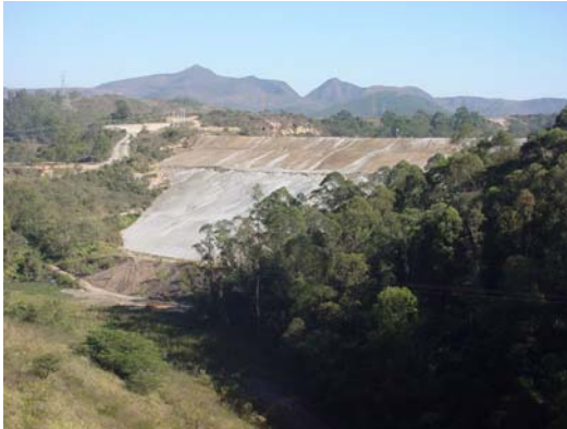
August 2002 - View of the impoundment wall at the start of rehabilitation efforts.
