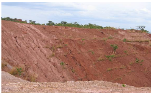
Vegetation planted on steep faces to control erosion.
