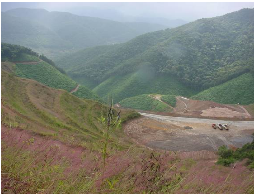
Pit slopes during rehabilitation efforts.
