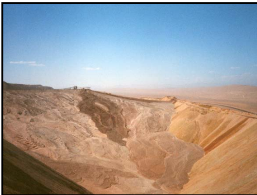
Figure 2.1.4: Filter cake disposal via conveyor in arid climate
