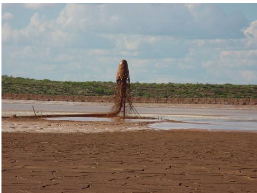
Central discharge point in basin of paddock/cell facility. Thickened tailings was used to change the slope from a concave to a concave profile to maximise capacity and form a shedding surface that is more amenable to closure.
