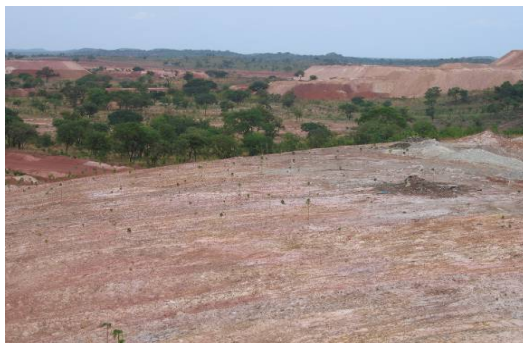
Waste overburden dump area reshaped and prepared for rehabilitation.
