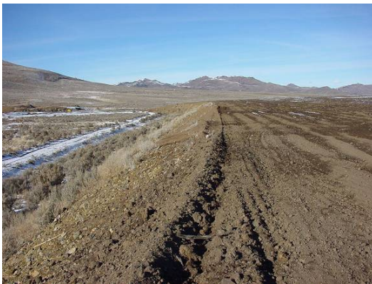
Crest of impoundment wall of tailings facility shortly after reclamation.
