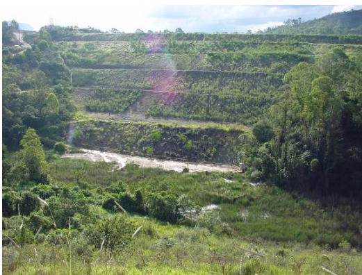
May 2004 - View of outer face of impoundment wall showing results of vegetation establishment programme.
