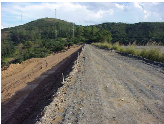
May 2004 - View along the impoundment wall crest showing clearing and earthworks for the next raise.
