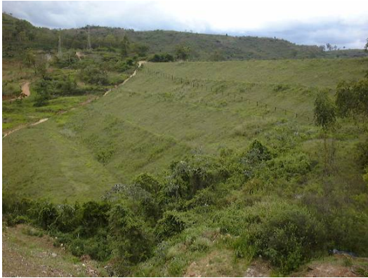
November 2001 - View of the outer face of the impoundment wall. Note the benches and grass-cover slopes.
