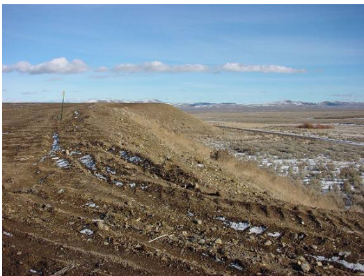
Outer slope of tailings facility.
