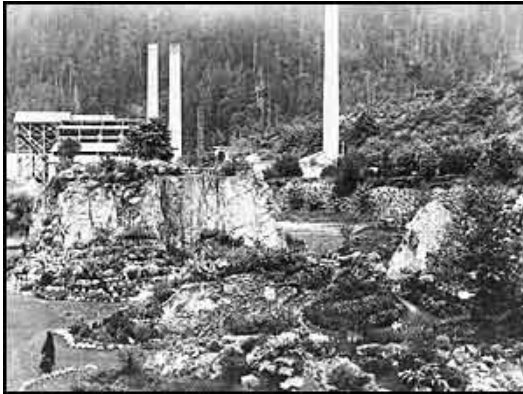
Portland cement factory at Tod Inlet on Vancouver Island.
