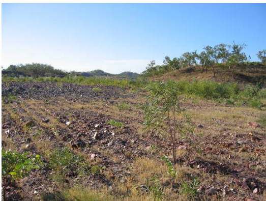
Waste overburden material and vegetation establishment on tailings facility basin.
