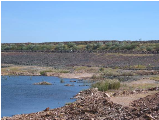
Main impoundment wall of tailings facility.
