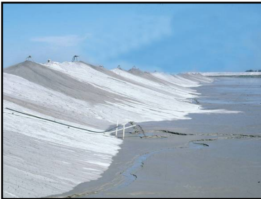
Figure 2.1.2: Tailings deposition behind a ring-dyke formed from the coarse tailings fraction
