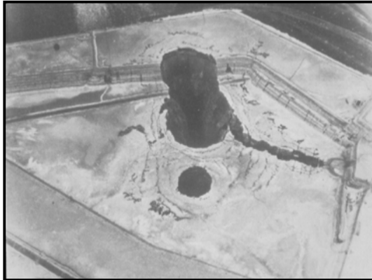
Figure 2.2.7: ARD at the toe of a tailings facility
