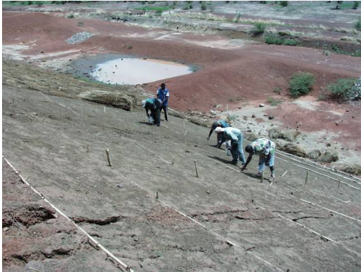
July 2002 – Compacted laterite starter wall seeding.
