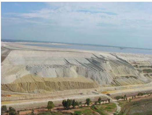
Rehabilitation trials with reshaping in progress.
