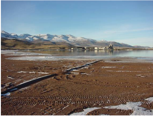
December 2000 – View of tailings facility showing reduced supernatant pool.
