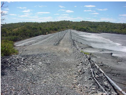
July 2003 – View along the crest of the impoundment wall – note the absence of vegetation.
