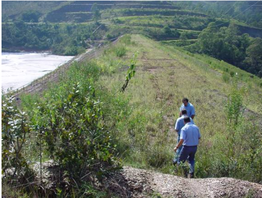
May 2004 - View along crest of the impoundment wall showing good vegetation growth. Upstream face not vegetated.
