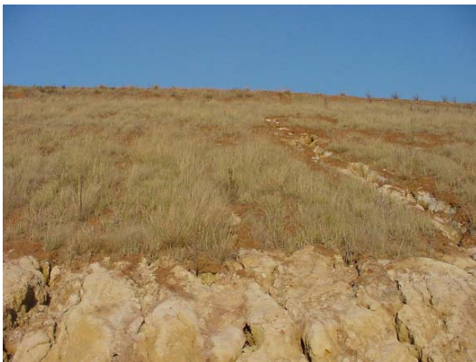
View of the face of the tailings facility from the toe looking upwards. Note the erosion channels and the absence of vegetation close to the toe.
