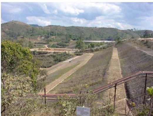
July 2003 - View along benches showing neat profile and successful vegetation establishment.
