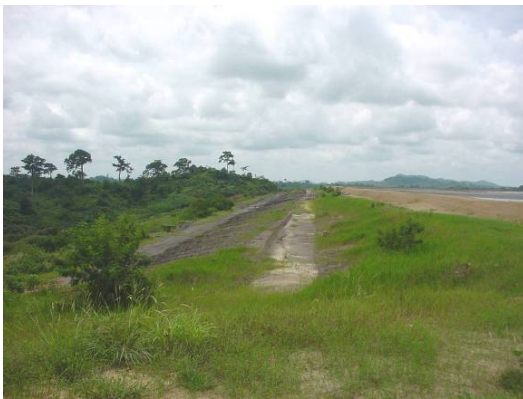
Sansu tailings facility – progressive rehabilitation of outer slopes.
