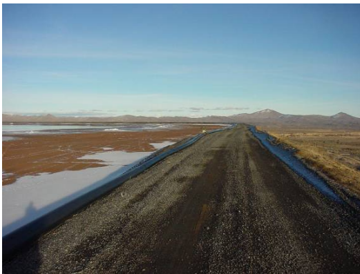
December 2000 – Crest of impoundment wall.
