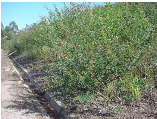
May 2004 - View of toe of bench showing vegetation and storm water collection channel at toe.
