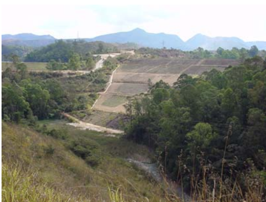
July 2003 - View of impoundment wall with rehabilitation efforts evident.
