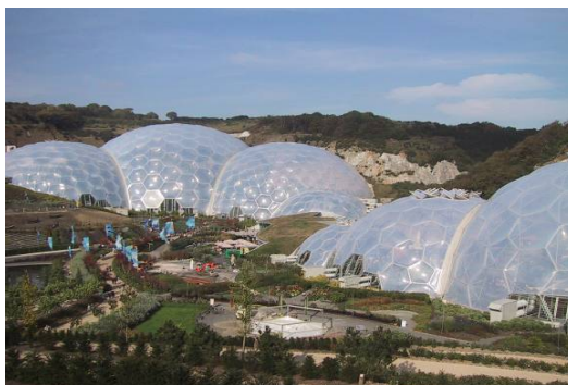
The completed biomes.
