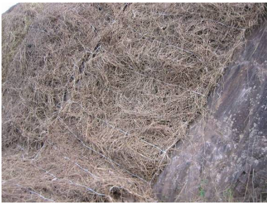
Wooden pegs used to secure pegs to high wall face.
