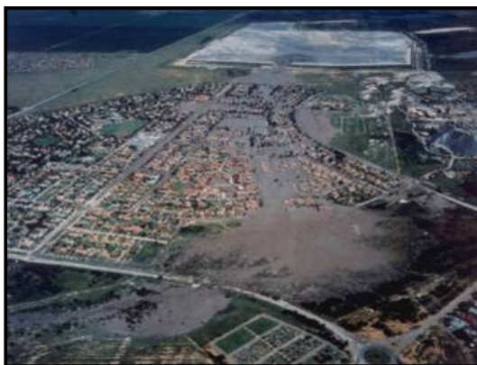
Figure 2.2.3: Merriespruit slimes dam failure in 1994
