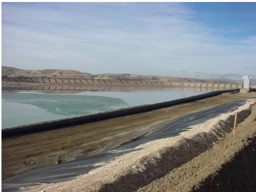
View over the basin of the tailings facility showing the deposition points around the perimeter.
