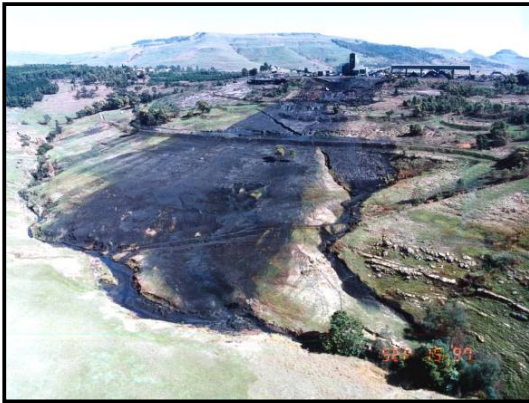
Figure 2.2.4: Colliery washing plant pond failure
