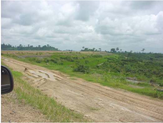
Sansu tailings facility – some revegetation of outer slopes during operational life.
