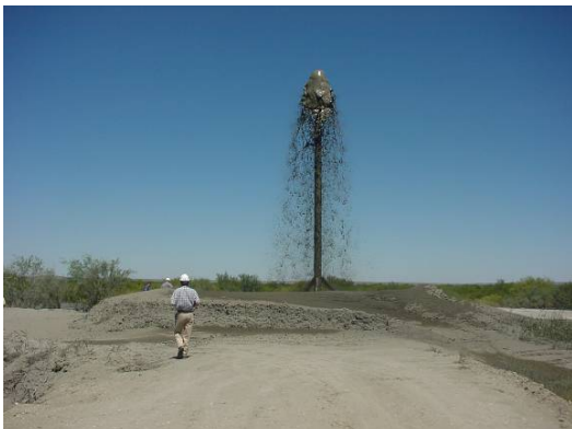
Thickened tailings discharge stack at tailings facility.
