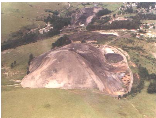
Dump D during rehabilitation.
