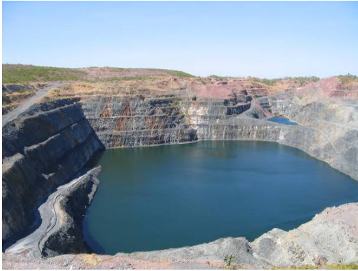
Disused pit containing tailings.
