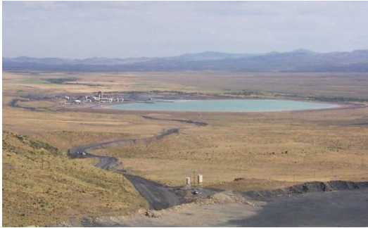
August 1999 – view of tailings facility showing the substantial supernatant pool.
