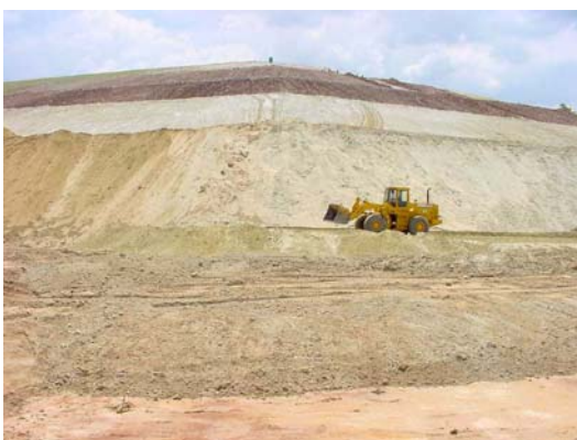
Reshaping and armouring of external corner (Windy Corner).
