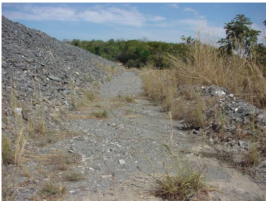
July 2002 – View along bench – note the good freeboard provided at the outer limit of the bench.
