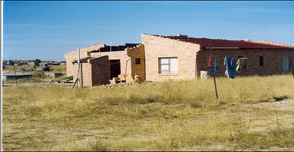
Figure 4.4 - pictorial view of Ha Tsolo settlement, Sealong. (A house built incrementally)
