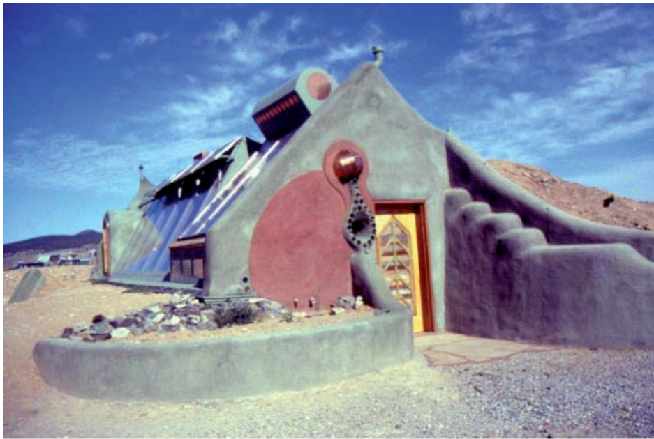
Figure 1d: Reynolds, M. (Mike Reynolds' own house in Taos New Mexico. http://www.independent.co.uk/environment/green-living/earthship-enterprise-the-ultimate-ecohouse-869591.html . Cited 30 May 2010.
