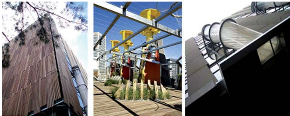
Images showing the operable timber slats, wind turbines on the roof and the shower towers on the north elevation.
