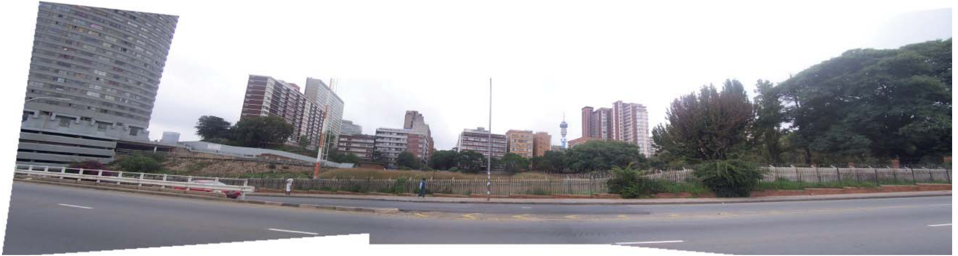
East elevation of site. (View from Joe Slovo Drive)
