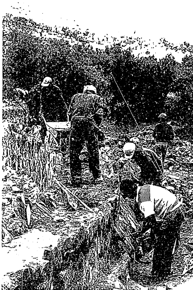
Fig 2.5 Typical division of tasks during the building of Bakubung Dam in the Pilarsberg Nature Reserve. The "skilled" labourer on the right is building outer leaves which will act as permanent formwork to contain the more fluid (inner) masonry which is being placed by the unskilled labourer in the centre.
