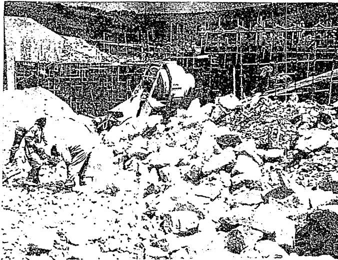
Fig 6.7 An inappropriately situated batching plant near the river bed level downstream of Maritsane Dam. Note the wheelbarrow haul ramp up to the work-face. The human energy cost of positioning the batching plant at the level of the foundations of a structure this size is estimated to be about 270 man days. A more appropriate position would be above (at a higher altitude) one of the abutments.
