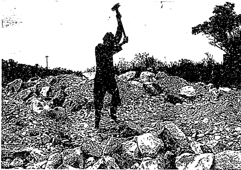
Fig 7.4 The practice of reducing the size of unwieldy granite boulders into manageable chunks with a sledgehammer is common in Zimbabwe and was successfully adopted during the building of Maritsane Dam in South Africa. The granite boulders break relatively easily. Eye protection for the labourers is essential.
