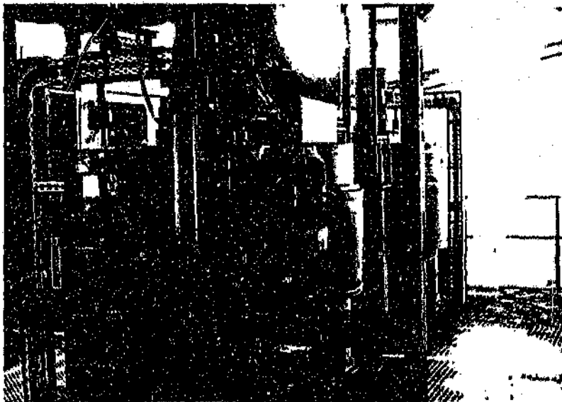
Photograph 8 - Mixer mill. Materials are gravity fed from the silos
