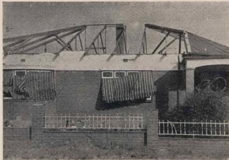
7. Trusses anchored to wall but purlins and roofing removed.
