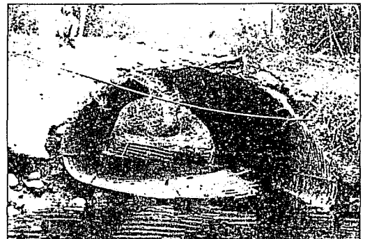
Fig 11: This corroded steel liner can be used as centring for a permanent RMC bridge replacement
