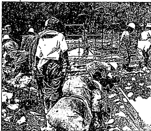
Typical labour-intensive casting of rubble masonry concrete (RMC). Here, a massive thrust block for the Maritsane Dam in South Africa is being built. The typical high proportion of mortar and the randomness of the rocks' shape, size and placement is evident in this photograph.
