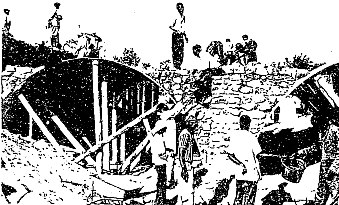
Fig 8.10 Cranked corrugated iron sheeting and gum poles used as centering in the Northern Province of South Africa.
