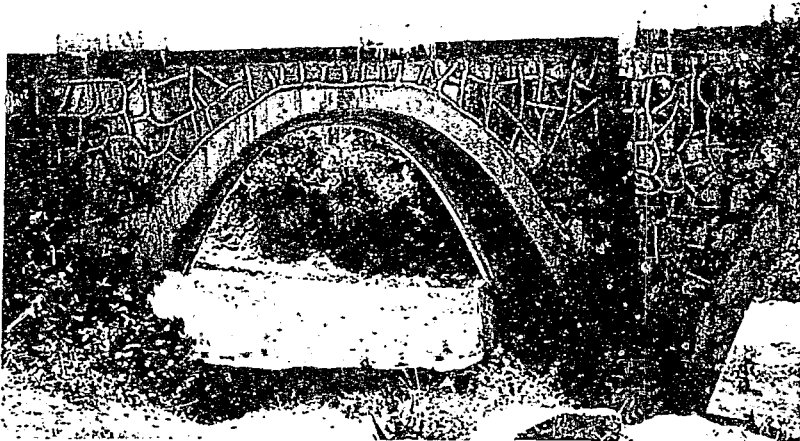
Fig 8.12 Proprietary precast concrete shells used as permanent formwork in Zimbabwe. The parabolic shape is highly efficient in minimising tensile stresses in the structure. Photograph courtesy of Fort Concrete Zimbabwe.
