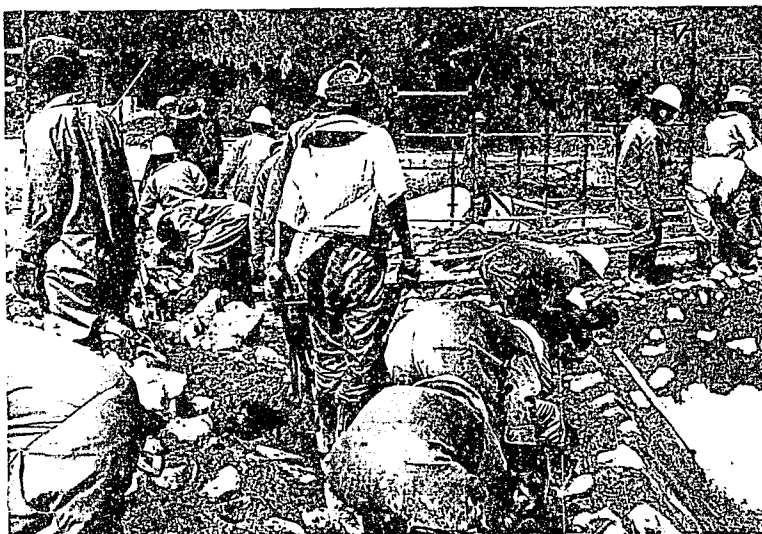
Fig 9.1 Congestion of labourers during the building of the thrust block of Maritsane Dam.
