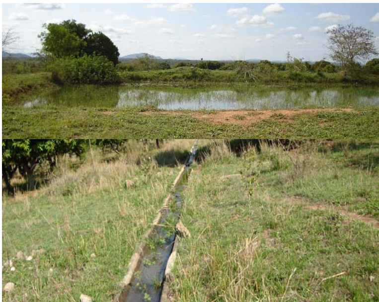
Figure 2.8 A lined irrigation channel leading to a night storage dam from an irrigation field.
