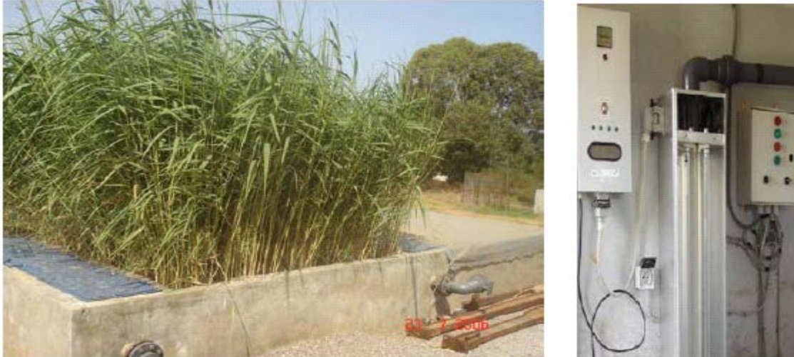
Figure 2.3: The reinforce concrete horizontal-flow gravel filter and UV disinfection unit
