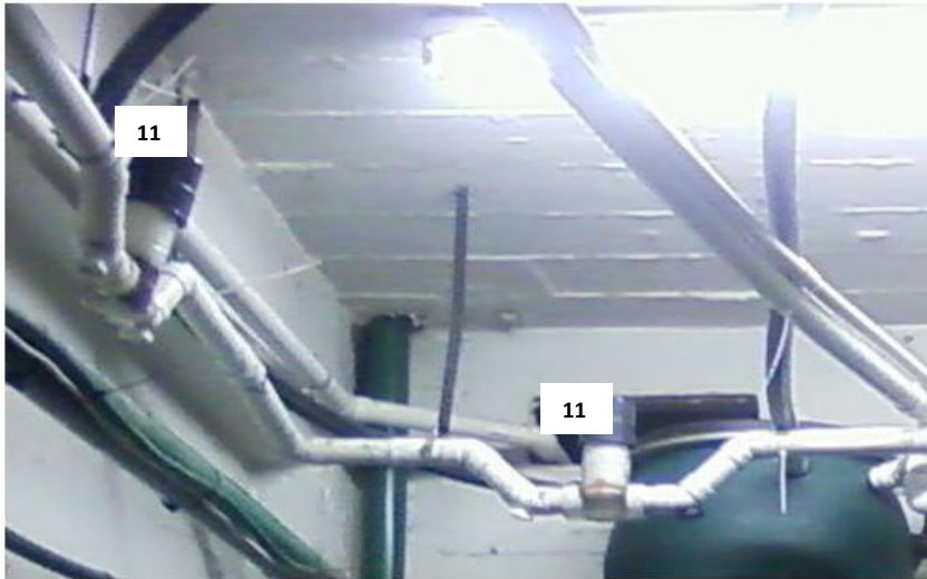
Figure 5.9. Inline chlorinators installed to improve disinfection of the greywater
