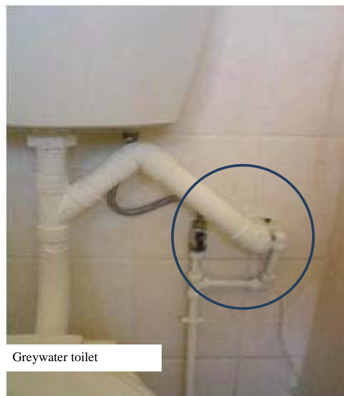
Figure 6.1b: The UJ dual potable and greywater pipe network showing the point of cross-connection located just before the greywater toilets (nodes 3 and 11 in Figure 6.1a)
