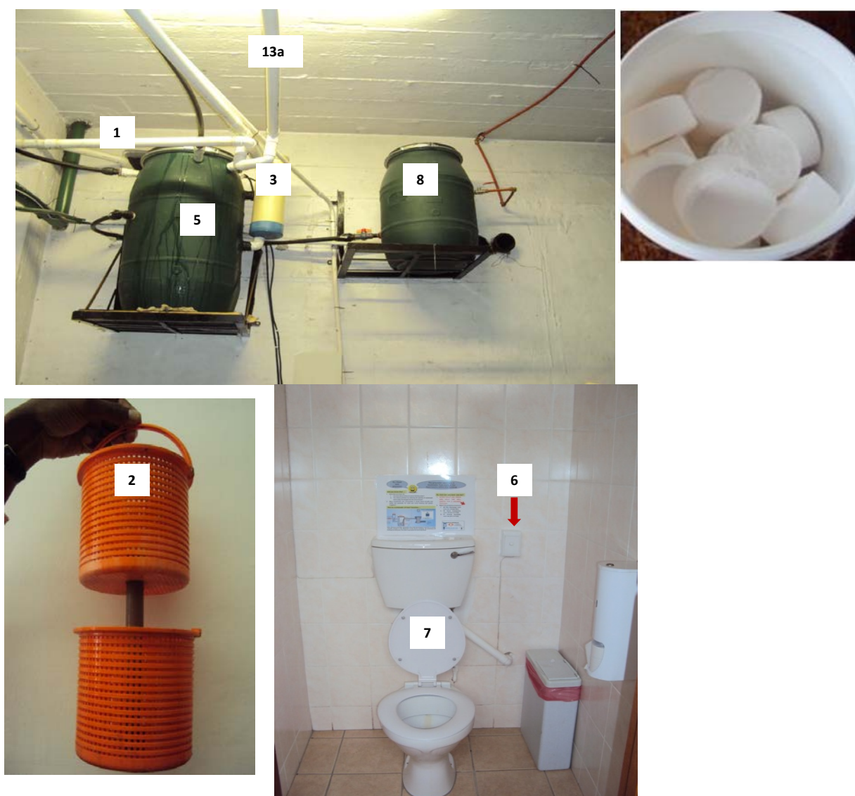
Figure 5.4 (a) The installed greywater (collection, sieving, pumping and storage backup) system (b) The 2 No. 2mm sieves used to sieve the greywater (c) Samples of the 200g Sanni Tabs (d) The female toilet connected to the greywater system
