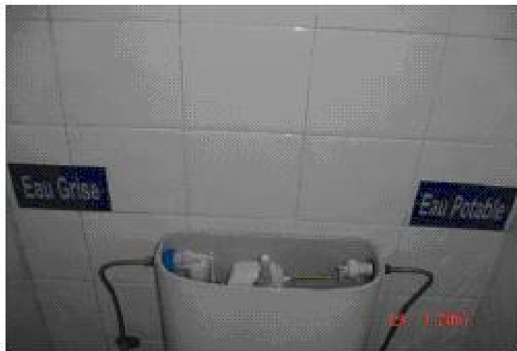
Figure 2.4: Dual piping supplies for toilet flushing
