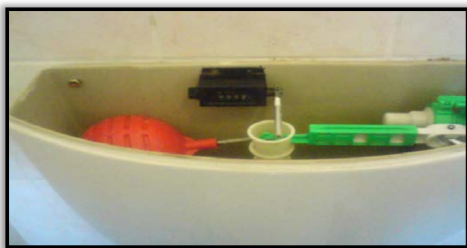
Figure 5.12: A displacement counter installed within a toilet cistern
