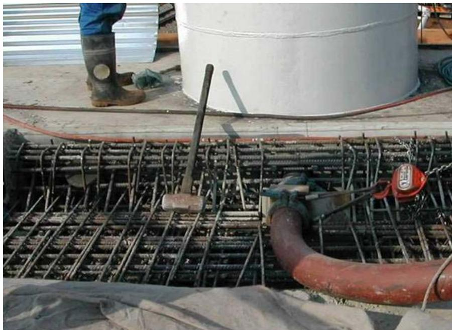
**Figure 2.2:** Pumping and valve arrangement at the pylon base<sup>(11)</sup>
