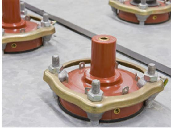
**Figure 16: Elastimold bushings as found on the hexa-transformer lid**
