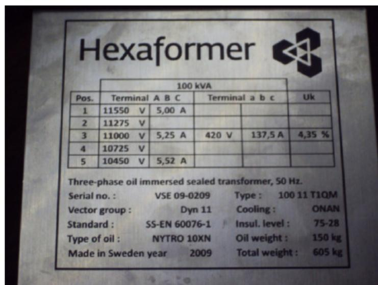
Figure 18: Hexa-transformer nameplate details
