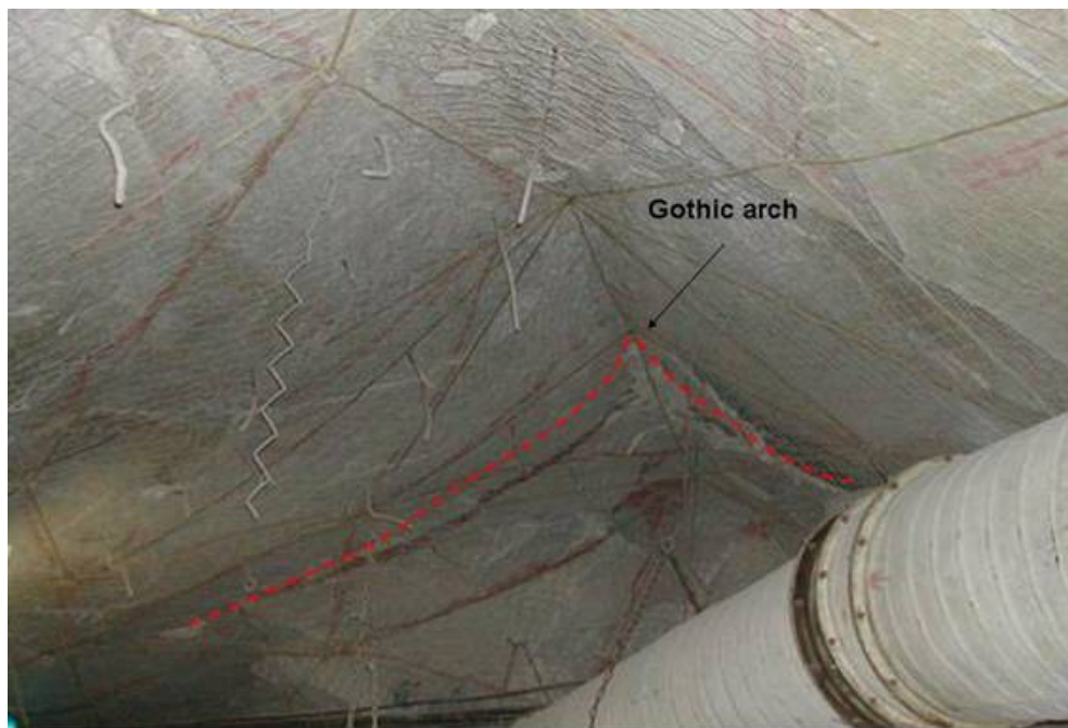
Figure E 58 Gothic arching in the 17 South Drive
