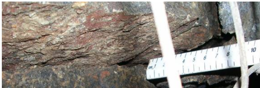
Figure E 11 Movement on a structure in the footwall during the mining of Panel 8s
