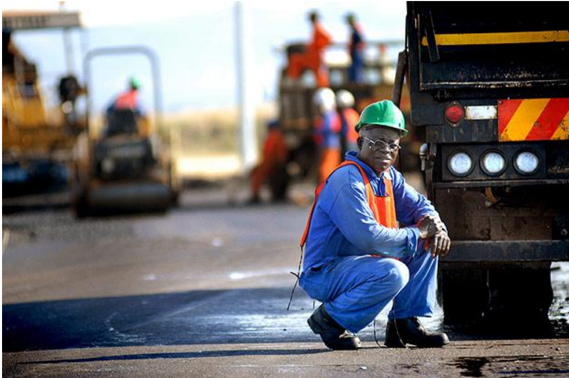
Picture 5-2: Road maintenance in Phokeng*
