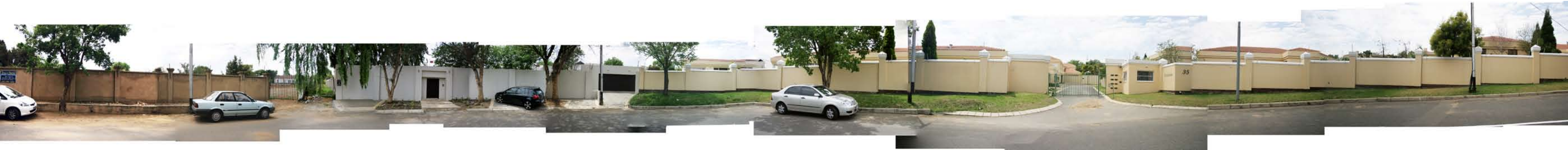
given more prominence than pedestrian access. Walls crowned with electric fencing obscure, if not eliminate, any views to or from the residences. Neat, well kept pavements, freshly painted walls and large trees and shrubs maintain the ambience of a typical older established northern suburb in Johannesburg.
