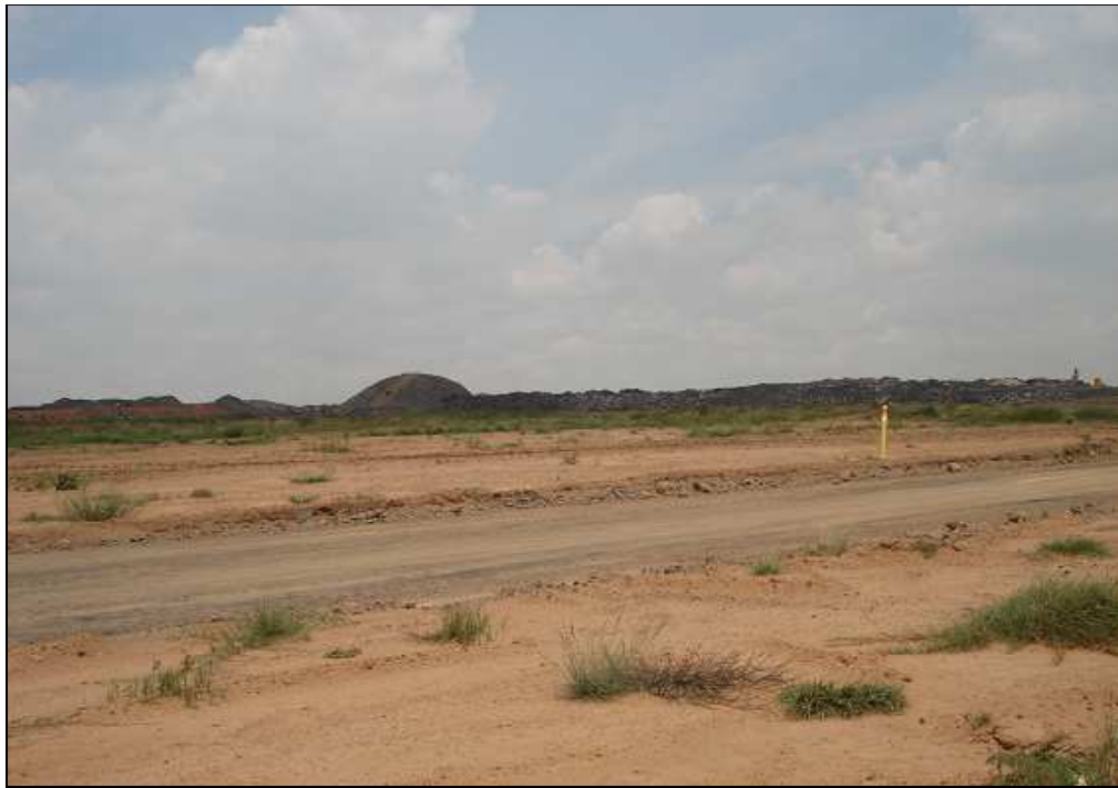
Figure 1.3: Photograph of Site Ramp 6 (South) at Schoongezicht Mini-pit
