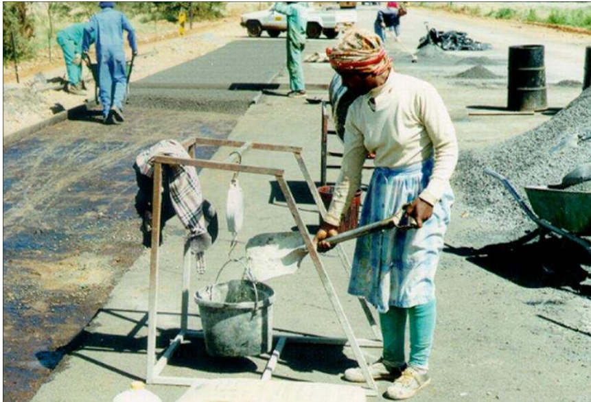
Figure 3.14: Labour-intensive construction of HVS test sections at Cullinan
