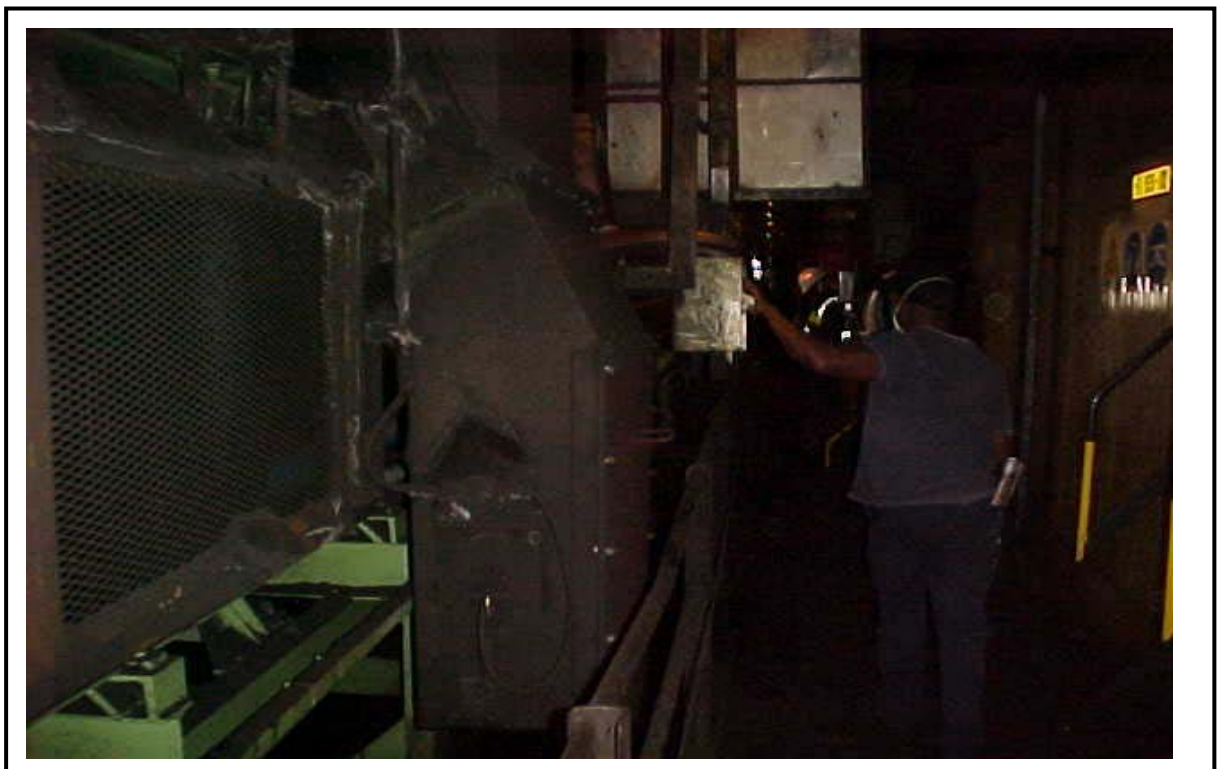
Plate 2: Tripper car operation
