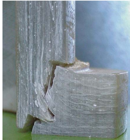
Figure 7.18: Crack extending through the flange radius
