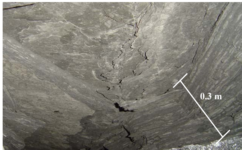
Figure 3.2: Photograph showing typical depth of gutter (about 0.3 m)
