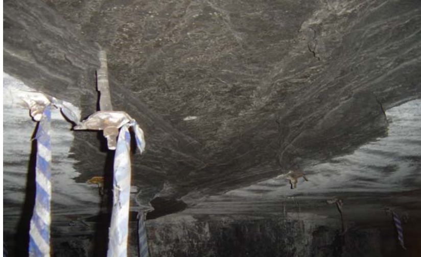
Figure 2.11: Guttering occurrence in a South African colliery
