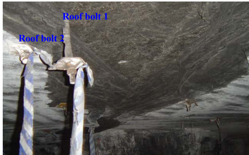
Figure 3.12: A roof bolt exposed due to guttering is replaced by another one
