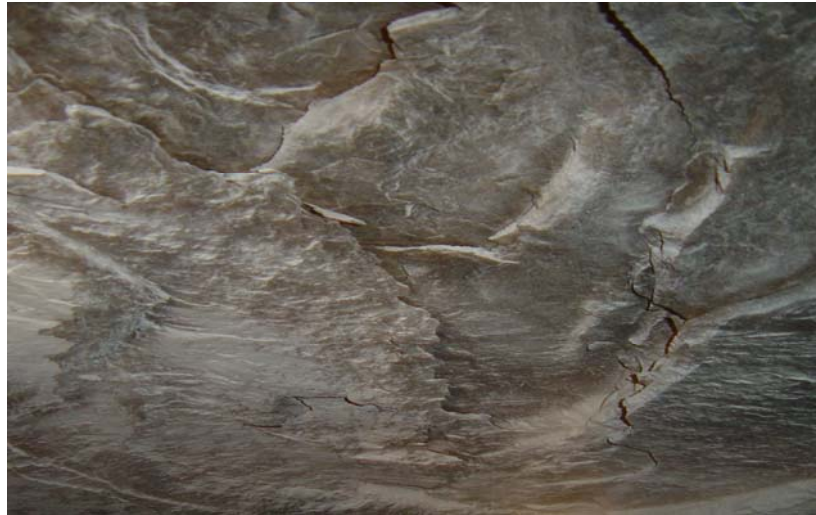
Figure 3.9: Interlocking nature of surfaces in guttering roof
