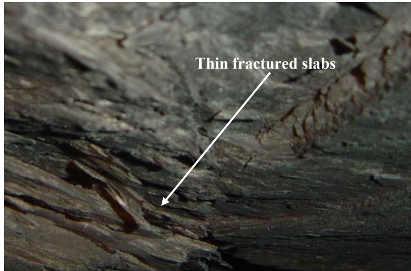
Figure 3.7: Photograph showing thin slabs associated with roof guttering
