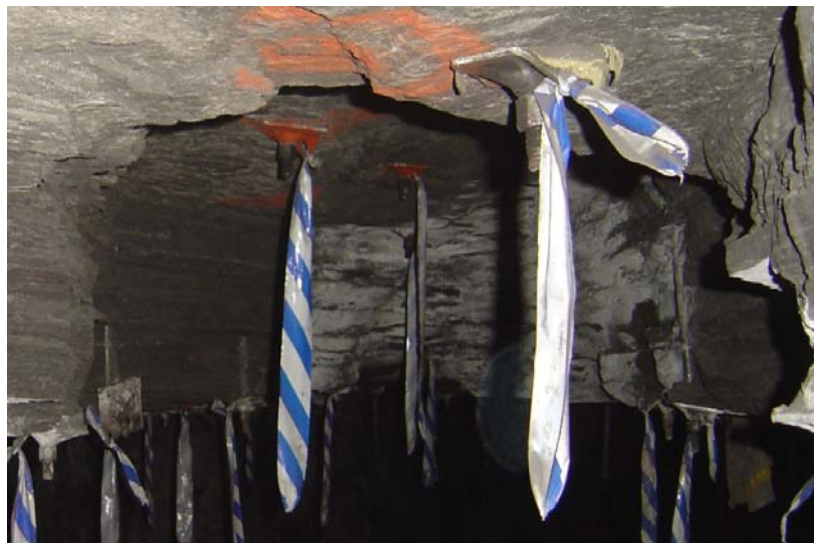
Figure 3.4: Photograph showing typical depth of gutter (about 0.5 m) and width of gutter (about 1.2 m)
