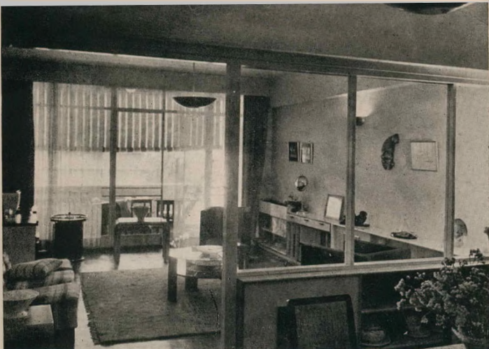
VIEW OF THE LIVING ROOM FROM DINING HALL OF FOUR-BEDROOM FLAT, showing glazed screen which defines these two spaces. The locally made light fittings are in spun unpolished stainless steel. The north wall is entirely of glass. Floor: Kiat block; walls, pale green and ivory; ceiling, white.
