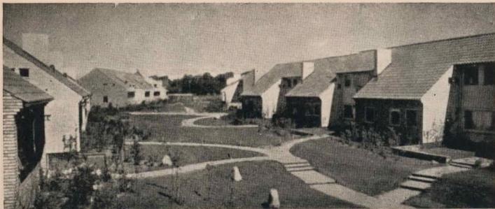
Swedish Row housing, with alternate houses back to front, creating private gardens. This illustration is of a very pleasant housing group, which, though the houses are of a fairly conventional design, they form part of a very small planned community.
