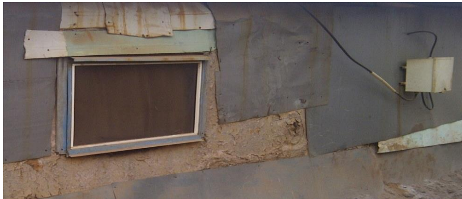
Figure 7: Electricity Access Point
