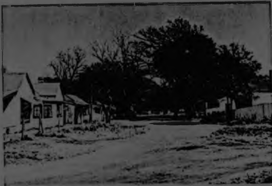
view to south east
