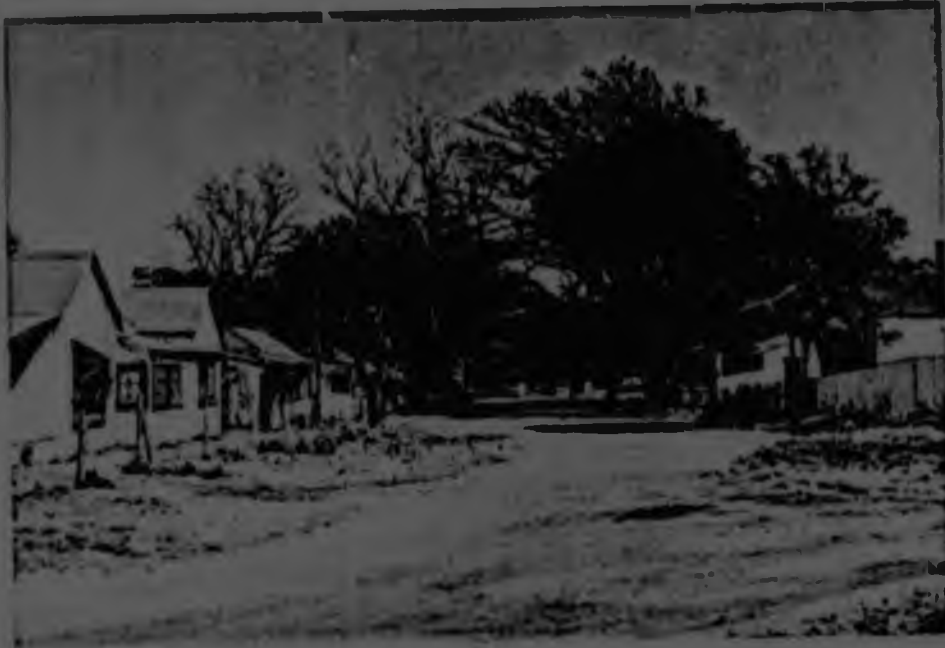
view to south east
