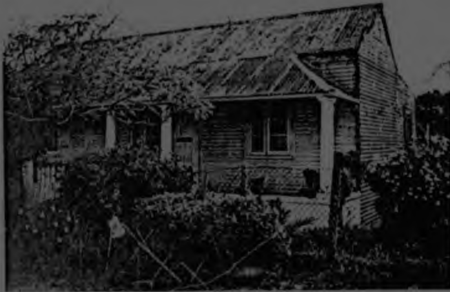
15 Wolsey Road note horizontal cladding
