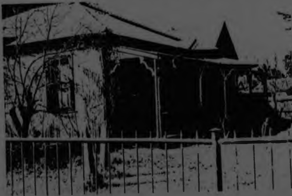
SIMMER & JACK MINES LIMITED Married quarters
