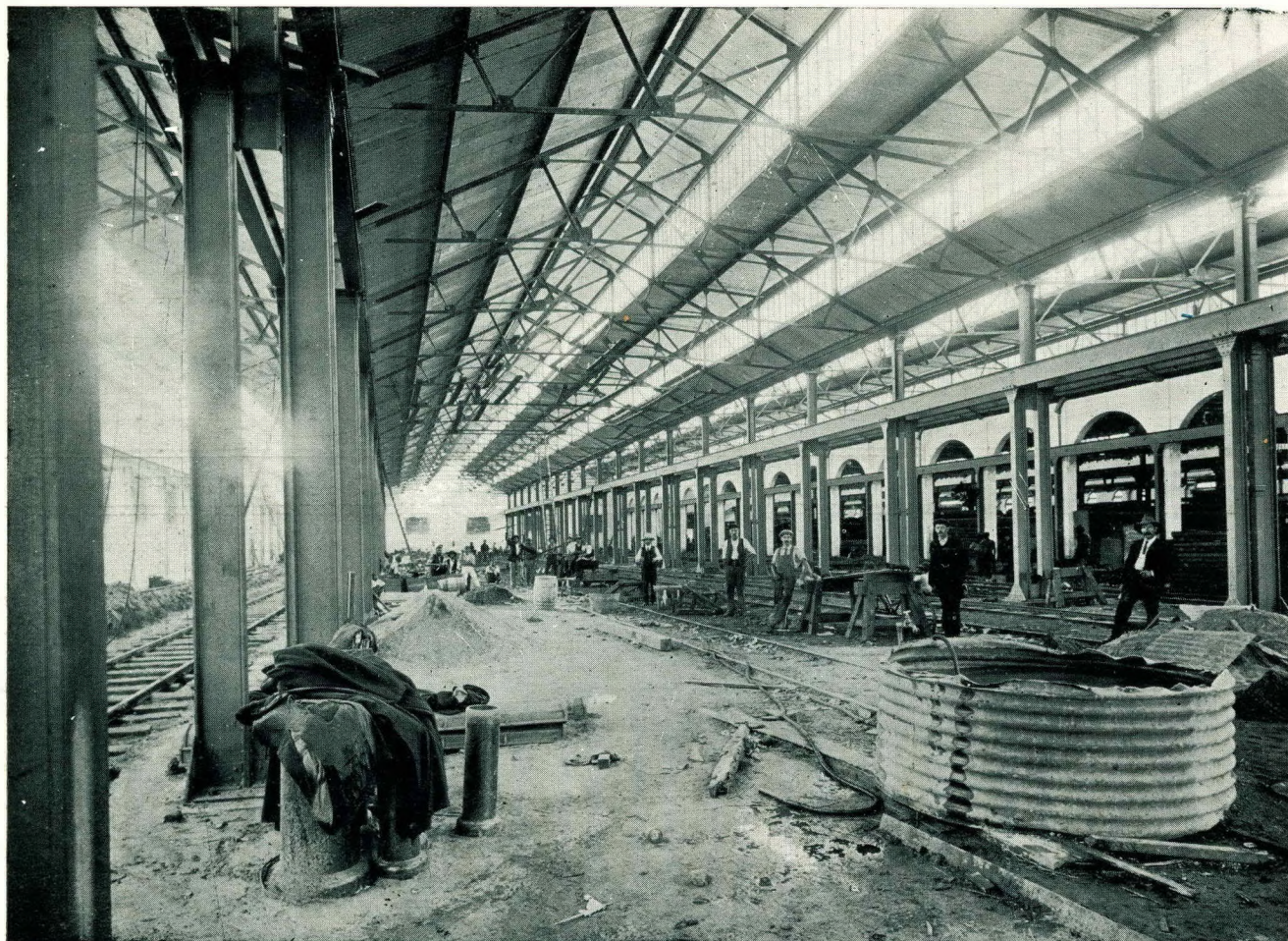
NEW CARRIAGE SHOPS, S.A.R., DURBAN: THREE BAYS, EACH 400 FT. LONG, 48 FT. SPAN, SUPPLIED AND ERECTED BY US COMPLETE.
