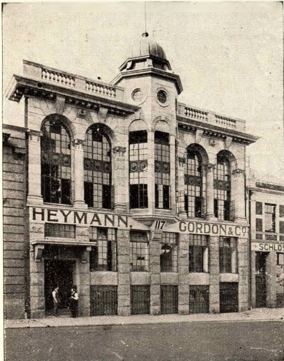
Reinforced Concrete Beams, Slabs and Columns on "KAHN" System Warehouse : Johannesburg
