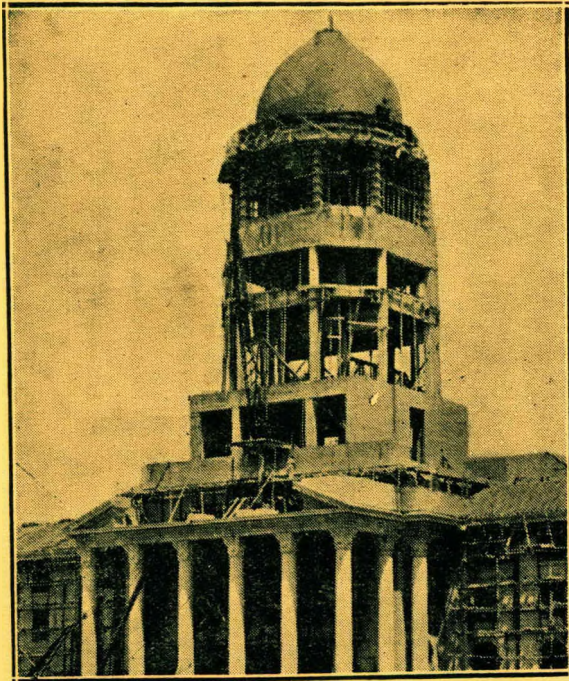
TOWER, NEW CITY HALL, PRETORIA.
