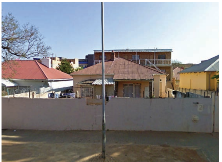
FIGURE 20: The flats behind this house have been built in the backyard of the property. No permission to build was sought. There is no way of knowing how safe the building is. There was also no opportunity for neighbours to object to an application to build. A policy is needed if such entrepreneurial initiatives are to be encouraged within a mandatory framework.
