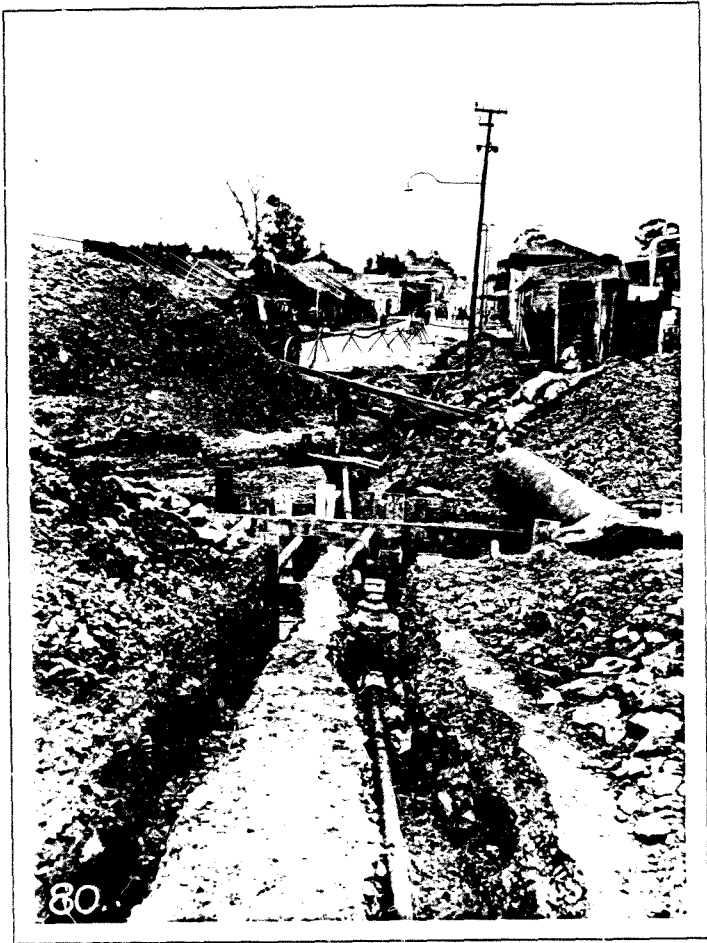
Water-pipe laying in Johannesburg, circa 1891.
