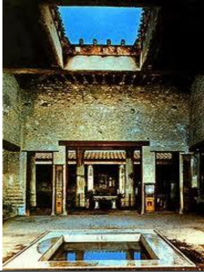
Fig. 12: An atrium at the House of Vettii, Rome, showing the area used for rainwater harvesting. Source: Study blue, 2012
