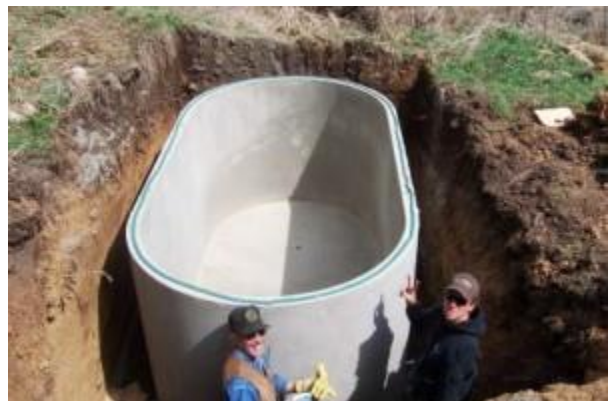
Fig. 20. A storage tank made of pre-cast concrete being advertised for use in Colorado. Source: www.westerngardeners.com
