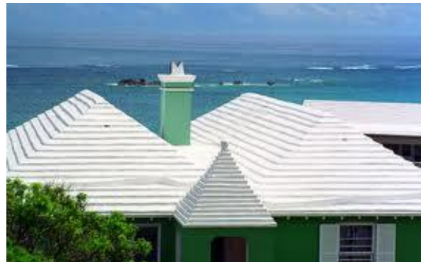
Fig. 22. A close up view of the horizontal grids on roofs that slows down speed of water flow Source: internationalchristianfictionwriters.blogspot.com.
