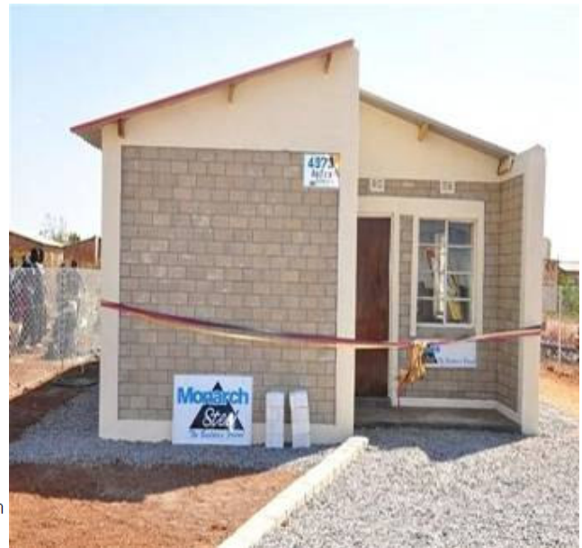
Figure 5(b): Typical Hydraform house completed
