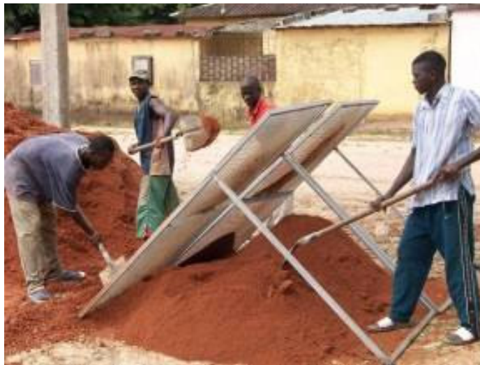
Figure 2: Sieving of soil for block production
