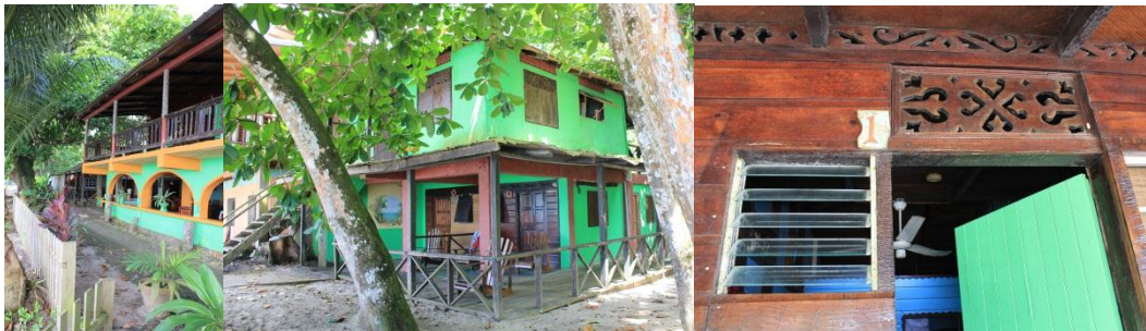
Figure 7.13. The buildings express the original hand-built design concept of Mt Plaisir the glass louvers however, are a recent addition, the windows used to have wooden shutters Source: Photographs by Daniella Sachs
