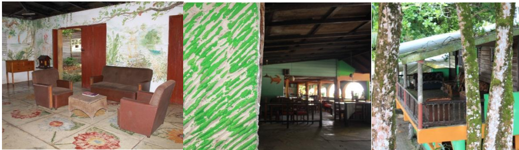
Figure 7.14. Traditional building techniques used at Mt. Plaisir include a decoratively coloured concrete floor, adobe plastering, and the use of wood cut in the “new moon” Source: Photographs by Daniella Sachs
