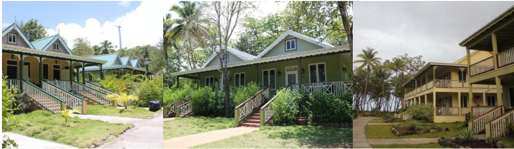
Figure 7.6. Rosalie Bay Caribbean-style cottages built out of reinforced concrete block with a stucco finish
