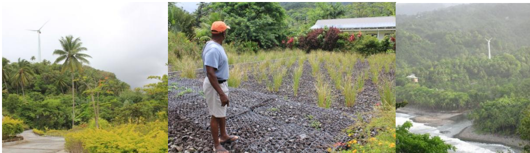
Figure 7.5. The Rosalie Bay wind-turbine towering above the forest; and the wetland sewerage system
