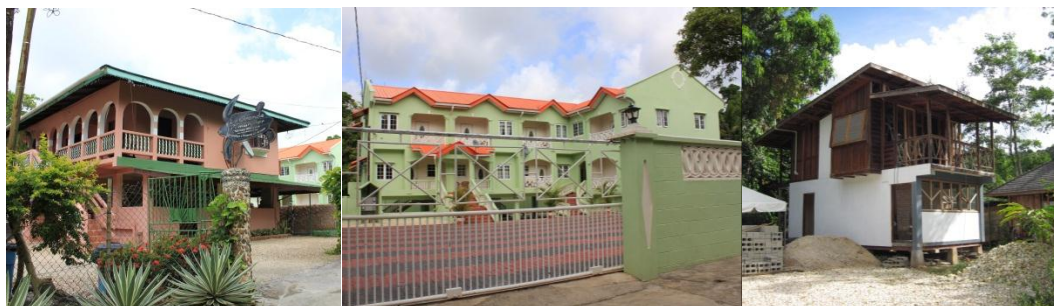
Figure 8.15. Grande Almandier Hotel and second phase condo development; Acajour construction of a new reception and office area Source: Photographs by Daniella Sachs
