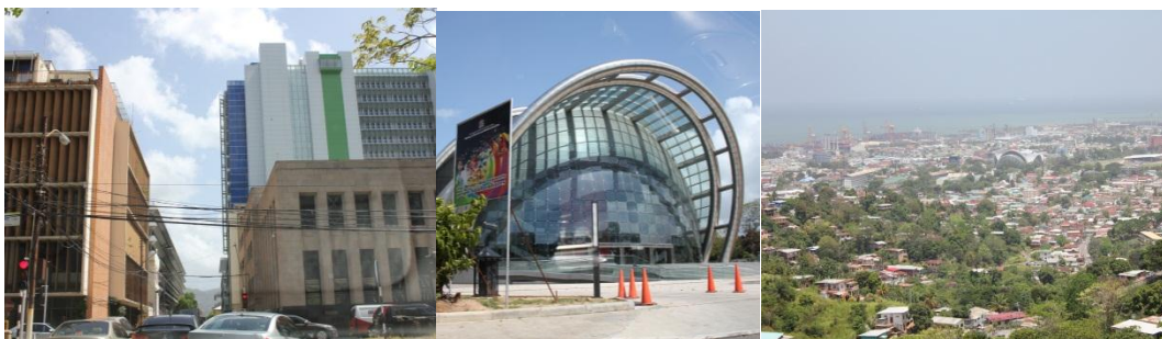
Figure 6.11. Downtown Port of Spain; the new Performance Centre; view over Port of Spain and the multiple building cranes
