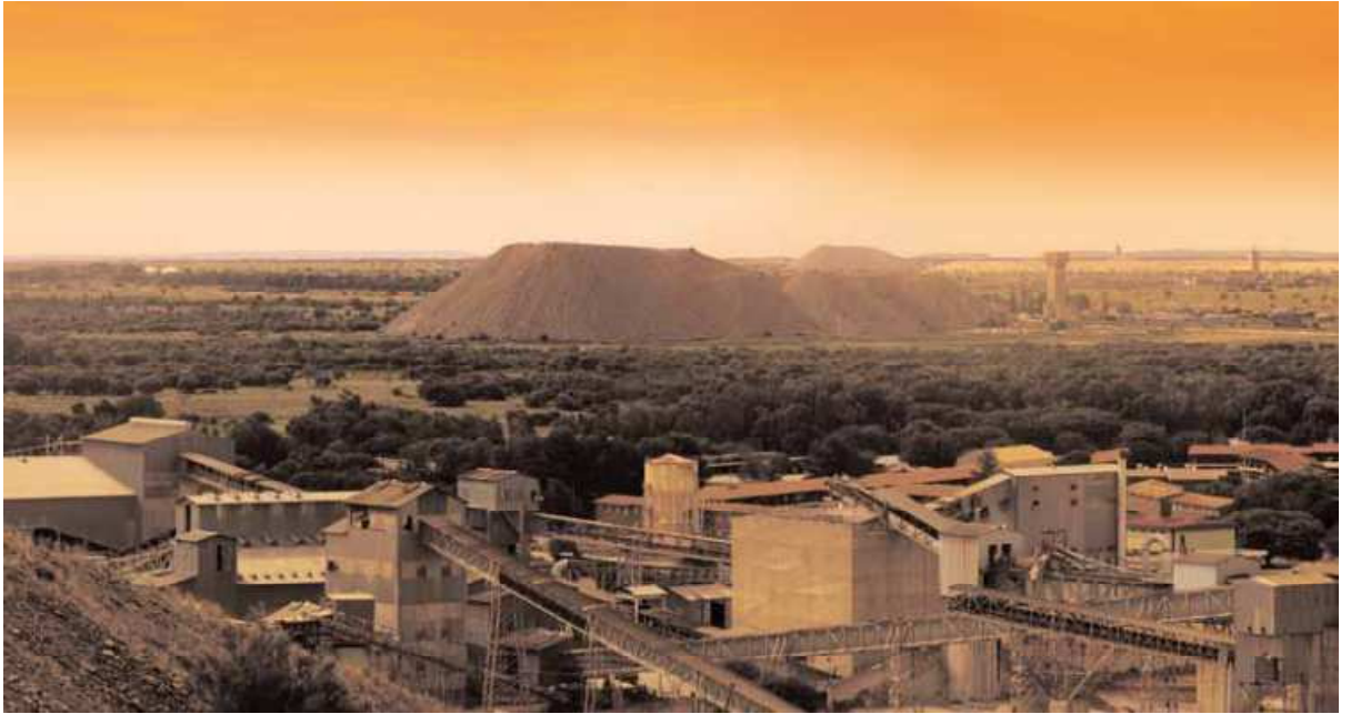
Figure 1.2. Photograph of a typical tailings storage facility (or tailings dam) (AngloGold Ashanti, 2007a).
