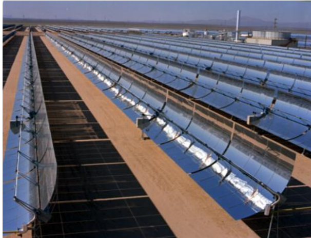
Figure 9: Solar trough plant design [12].
