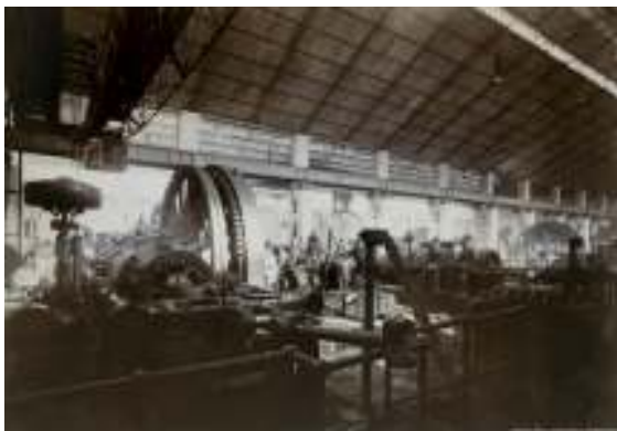
Image 4: Interior of the Electric Workshop (Johannesburg's first power station) – now Sci-Bono Discovery Centre
