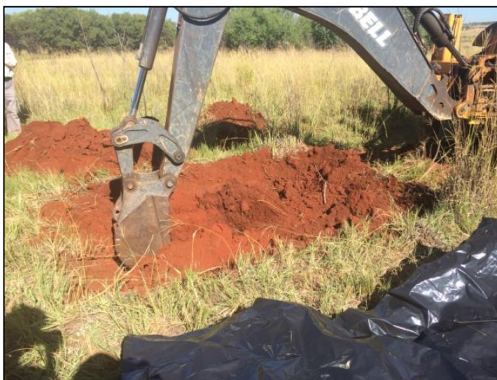
Figure 3.4. TLB in the process of removing soil from a Redsoils soil pit.
