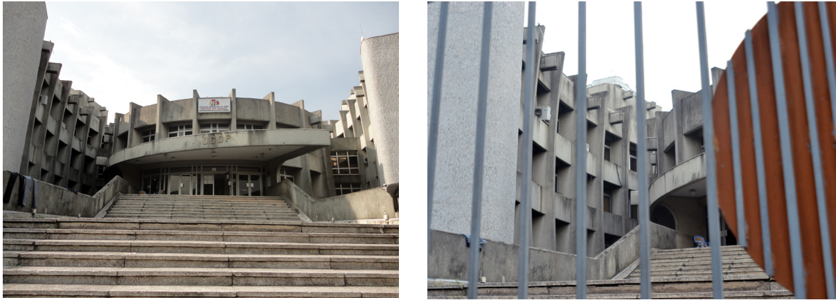
Figure 5.12: Contemporary image of OGEDEP (built in 1980)
